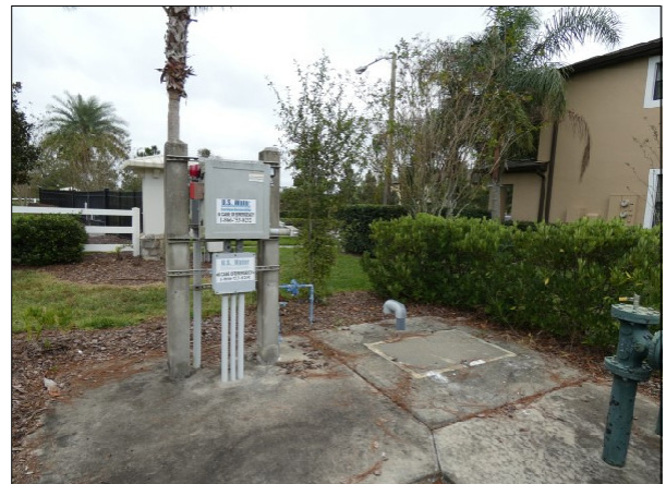
Meadow Pointe North Lift Station
