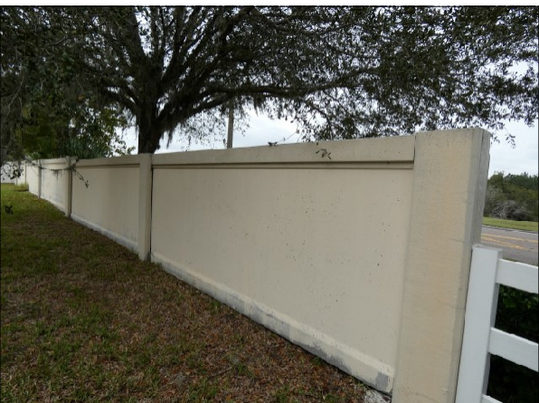
Parkmonte Masonry Wall
