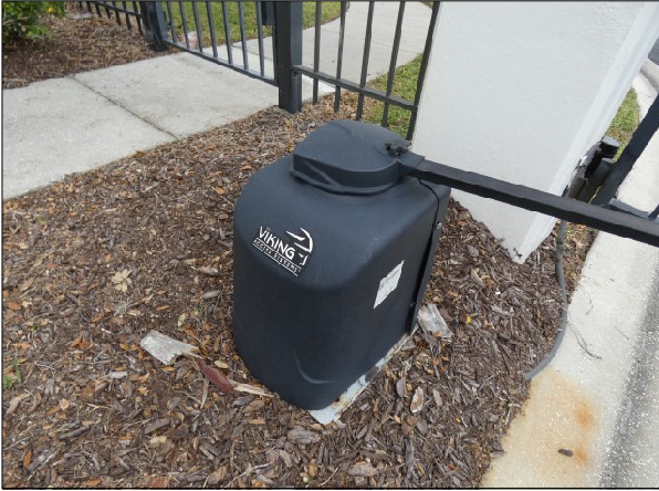
Typical Gate Operator
