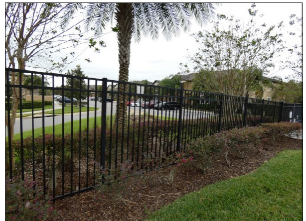
Typical Entry Aluminum Fencing
